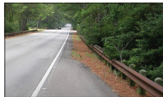
Add Metal Beam Guard Rails
