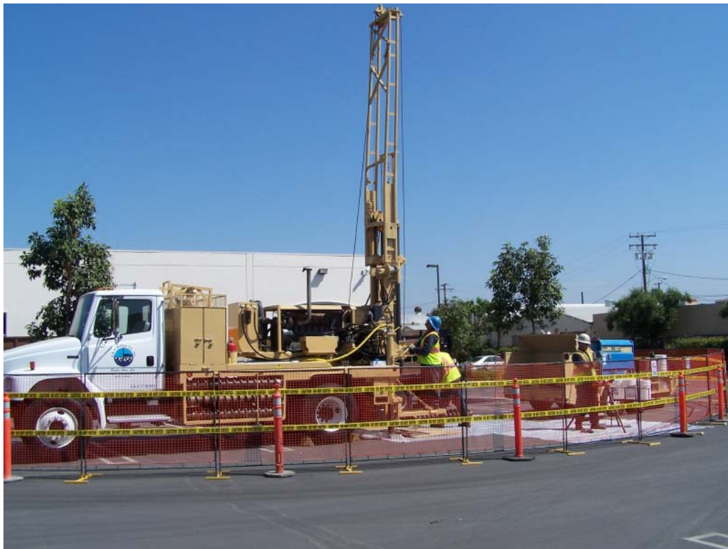
Example of a drilling rig
