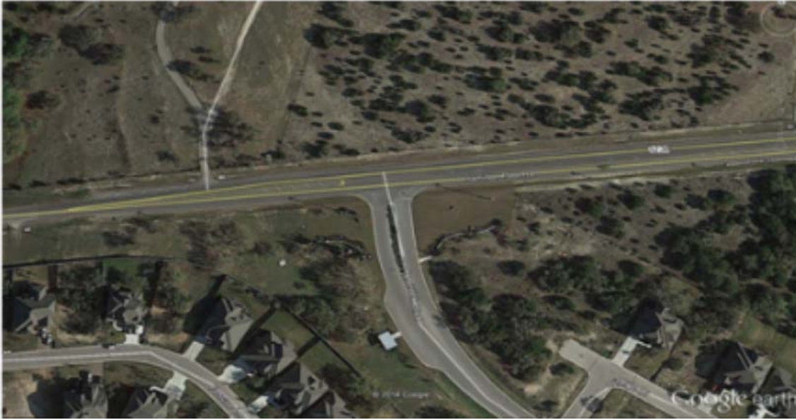
Example of a left turn lane similar to what will be constructed at the Crumley Ranch Rd intersection (photo of Rocky Creek Blvd intersection).
