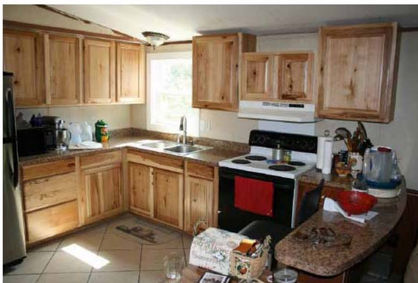
New sink, countertops, and cabinets
