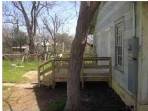
New electrical box and deck
