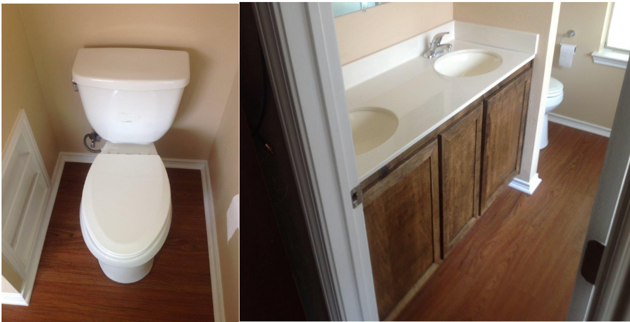
Before and after repairs of bathroom
