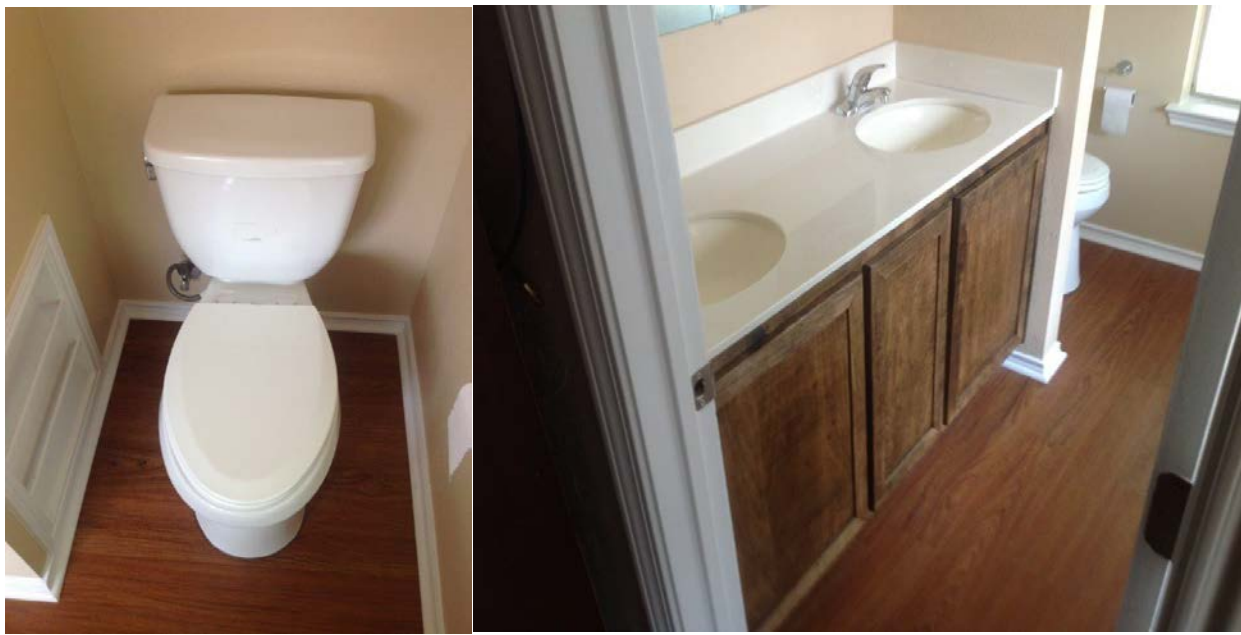
Before and after repairs of bathroom
