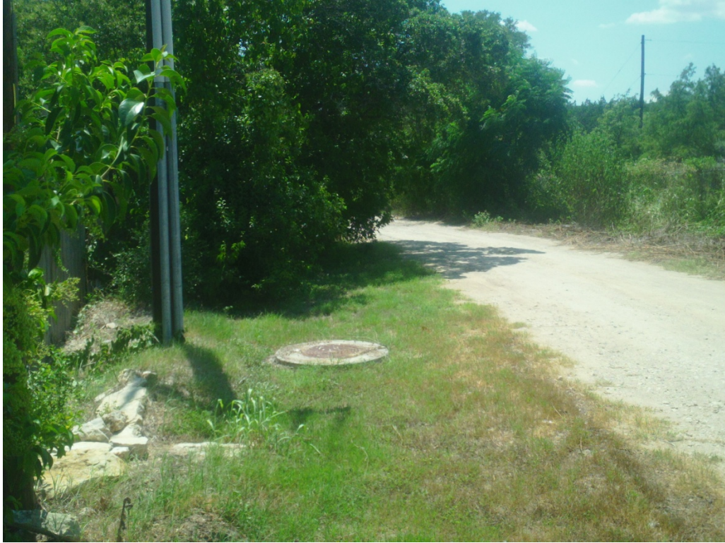
Photo 1: Overview of project area facing southwest down Meadowlands from Holly Lane.
