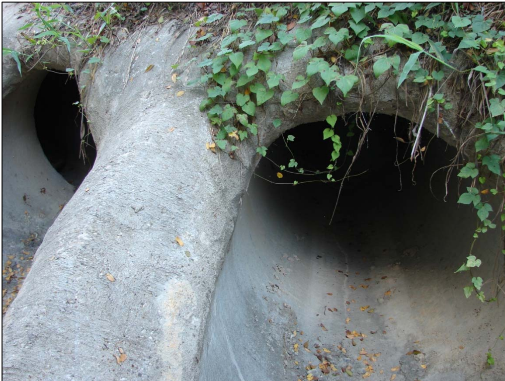
Photo 6: Culvert under North Meadowlark Street, facing northwest taken 9-21-2012
