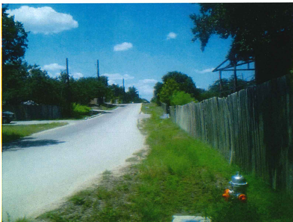
Figure 6: Overview of APE facing northeast from intersection of Covenant Canyon Road and Cavalier Canyon Road.
