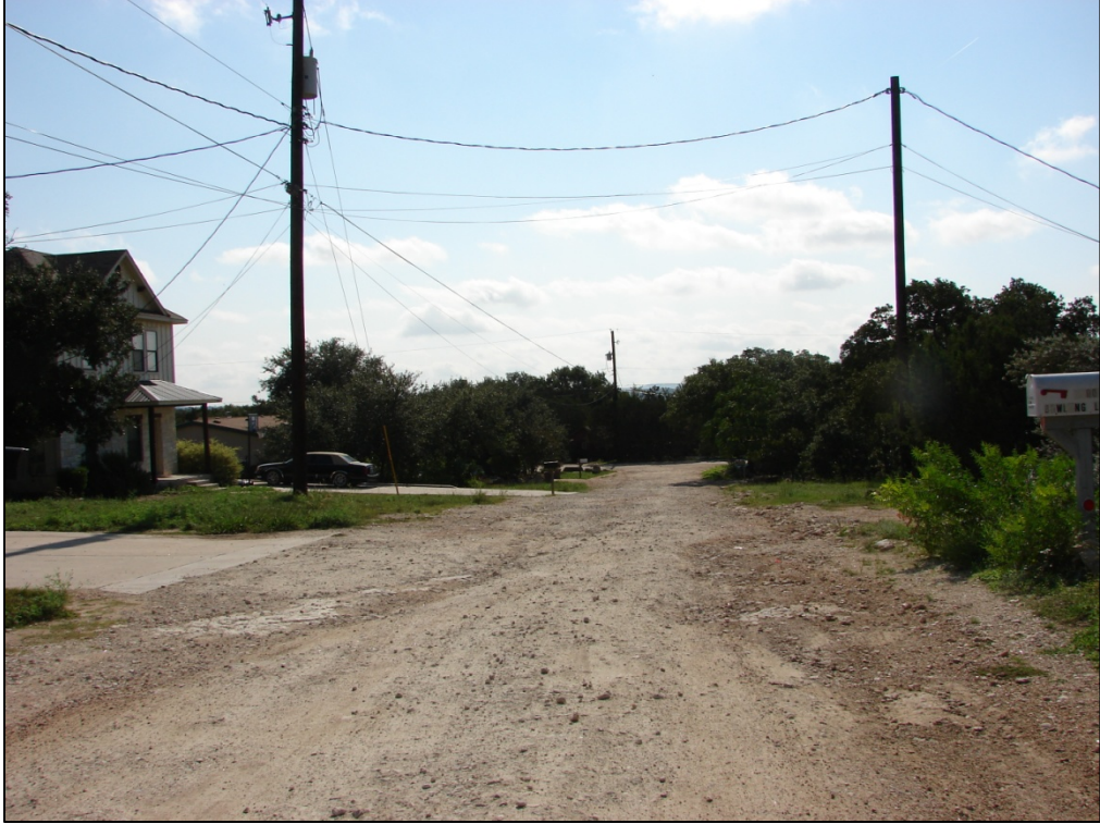
Photo 3: Bowling Lane, facing southeast taken 9-21-2012
