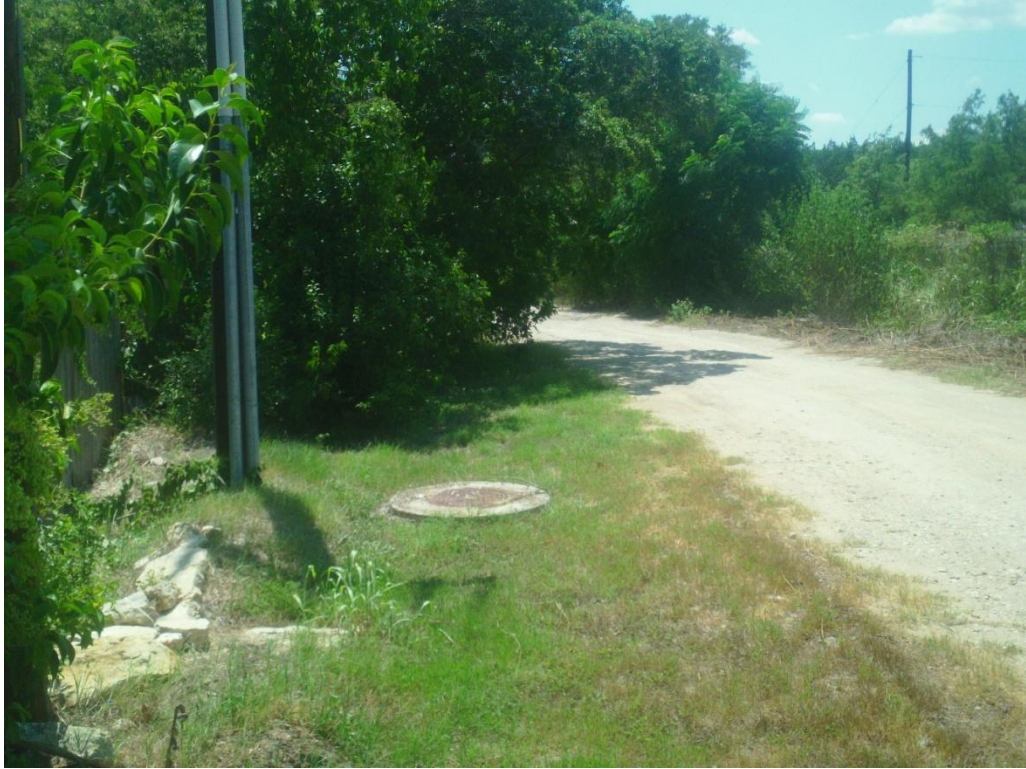
Figure 1: Overview of project area facing southwest down Meadowlands from Holly Lane.
