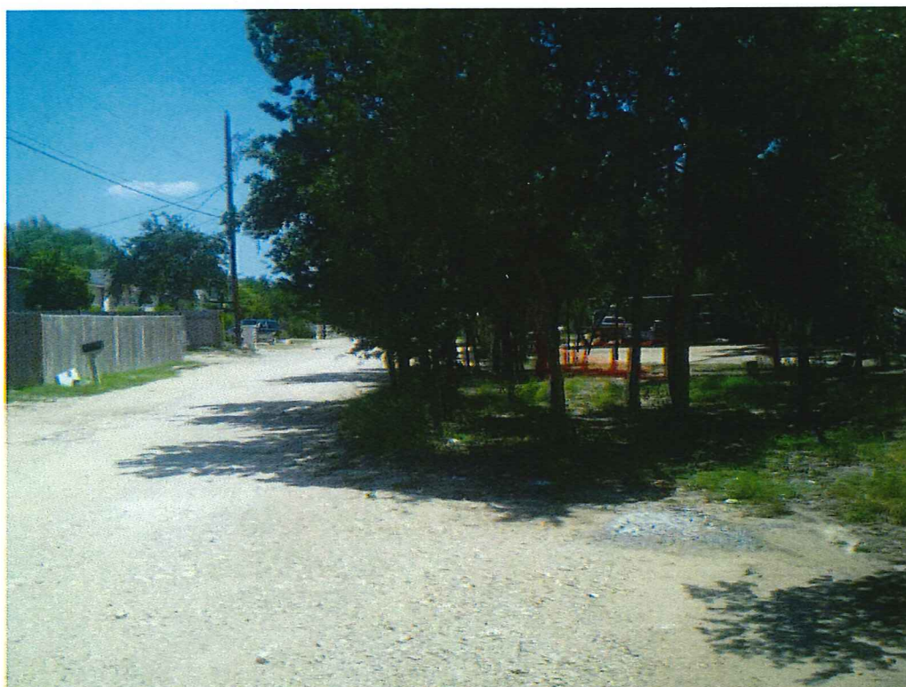
Figure 4: Overview of APE facing southeast along Holly Street.
