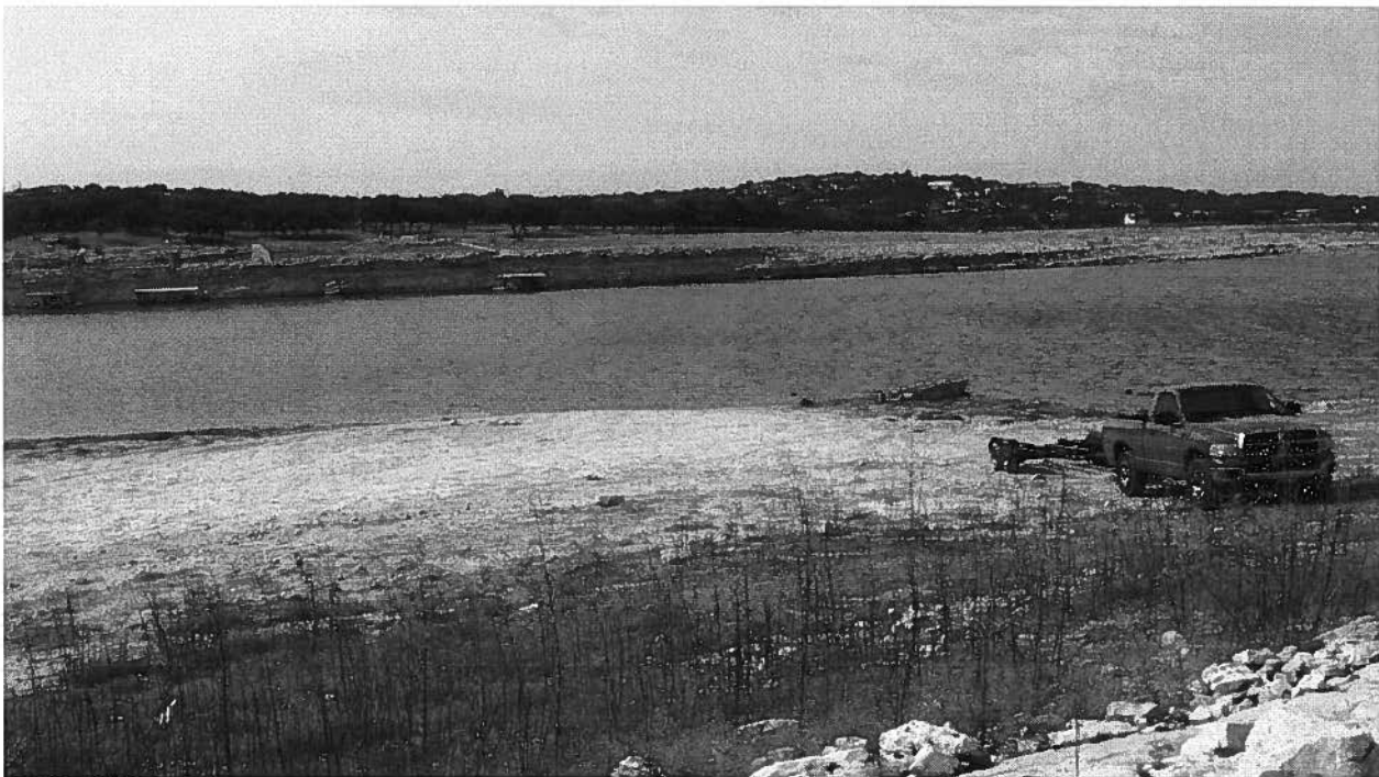
Photo of Tournament Point showing the proposed ramp location extending southeast into Lake Travis.
