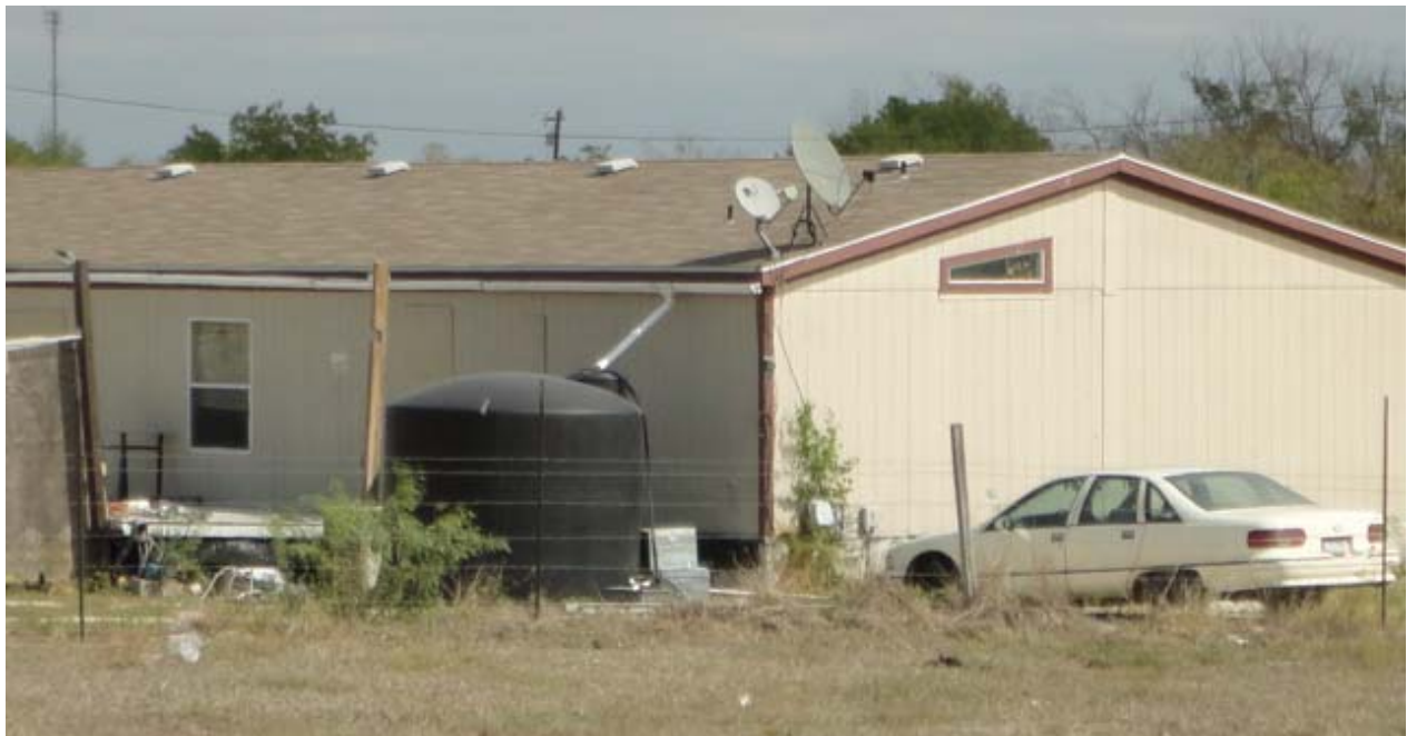
Water Storage and Pipe Connecting it to Structure
