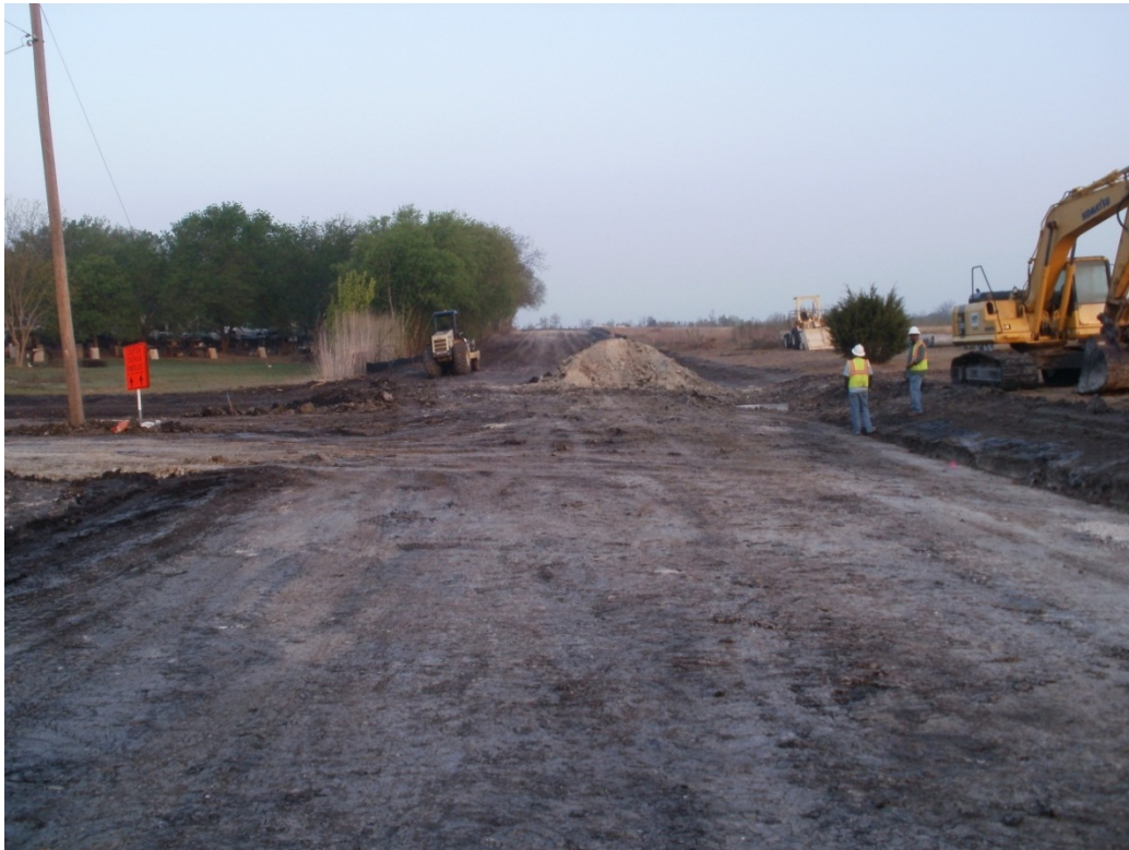
Lava Lane During Construction
