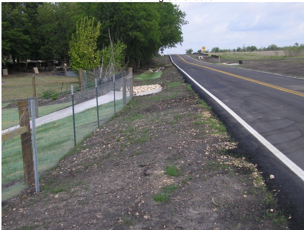
Lava Lane at Project Completion
