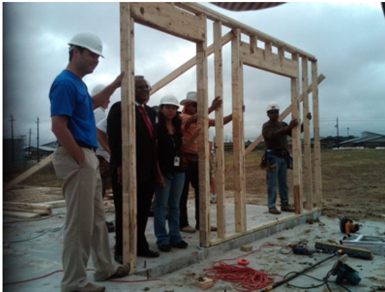
Wall-raising of first house for the project
